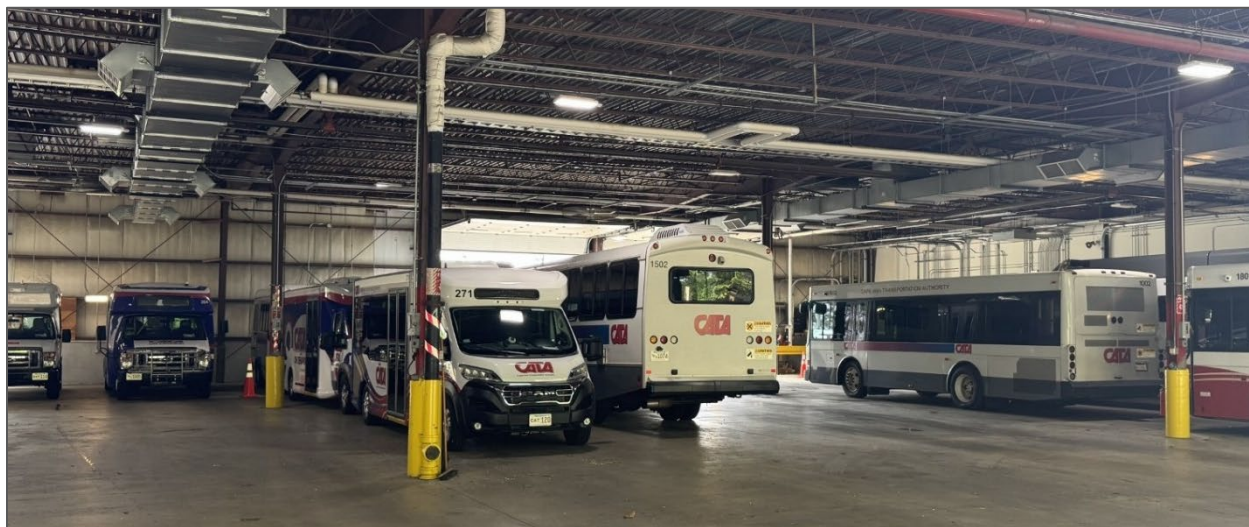
Figure 1. CATA Facility (Garage)
